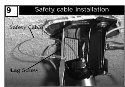
For Canadian installation and for USA fan and light kit combinations over 35 lbs, in both flush and downrod mode the safety cable must be installed into the house structure beams using the 3" lag screws provided. Make sure that when the safety cable is fully extended the leadwires are longer than the cable and no stress is placed on the leadwires.
